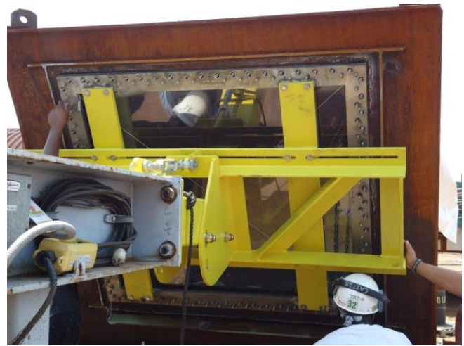
New fixture and process will improve TA window installation on aircraft carriers. NNS Photo
