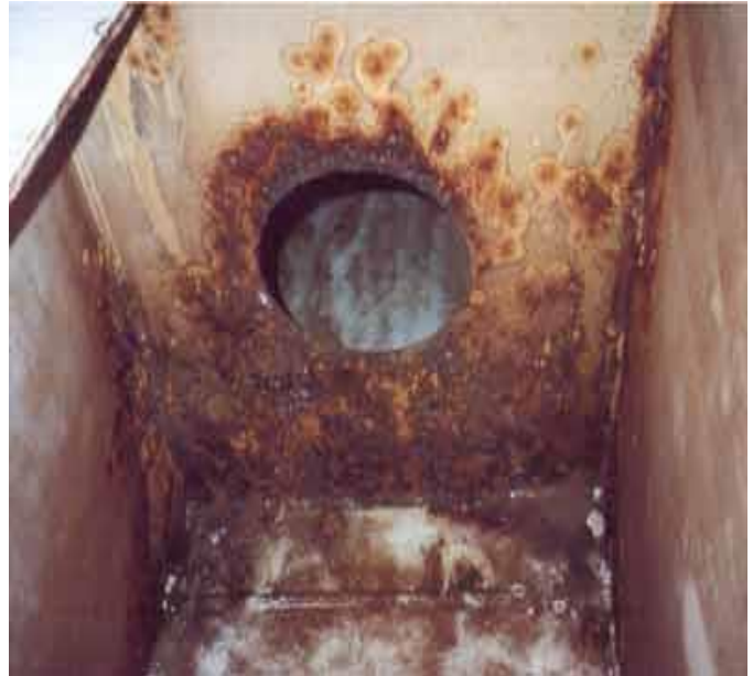
Mitigating surface contamination and efficiently controlling the environment to blast and paint CVN 79 tanks and voids could save cost and schedule risk.
