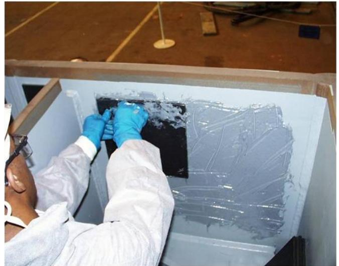
PMS 450 will validate alternate cost-saving damping adhesive that was identified in this NMC project. NNS photo
